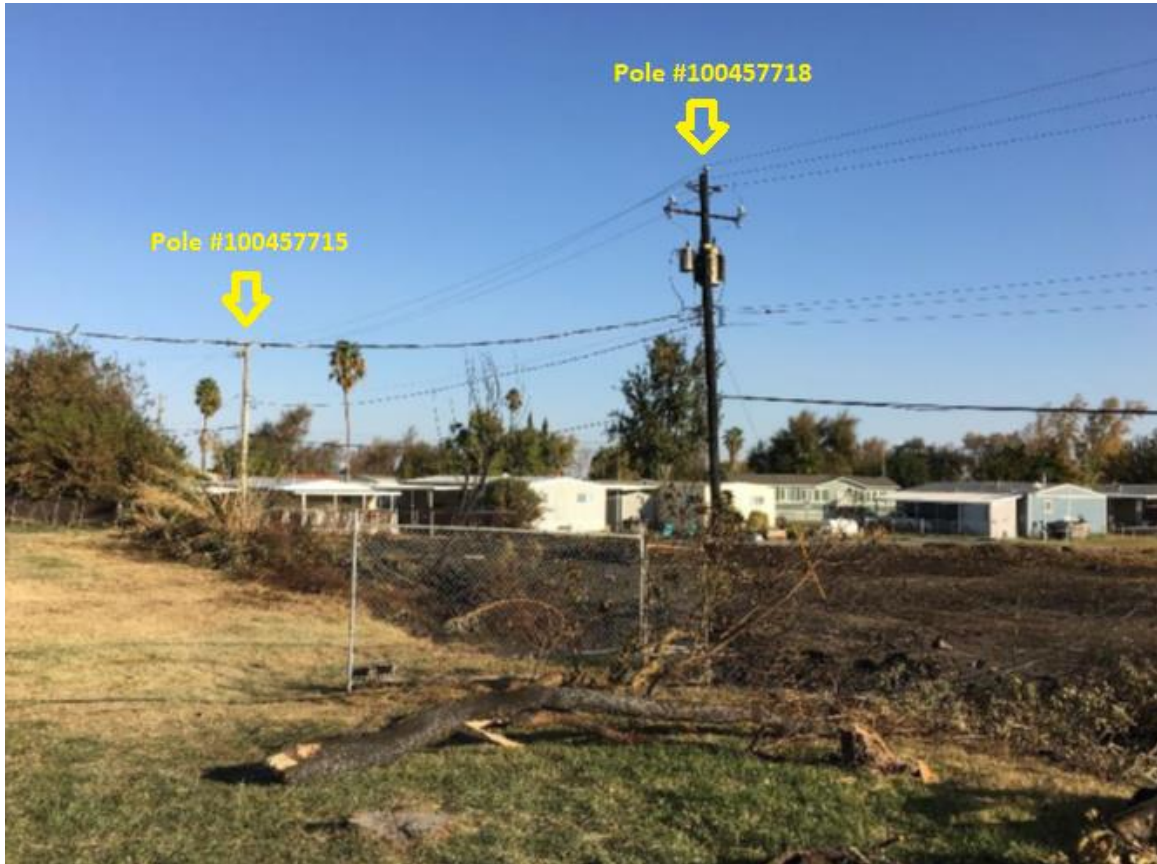
Figure 7: Charred field next to the Gateway Gas & Mart. Pole #100457715 is the subject pole where arc sparks were observed in the video clip shot by a witness at the time.
