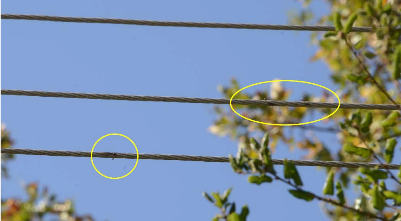
Figure 2. Photo showing broken/loose lash wire on communication cable.
