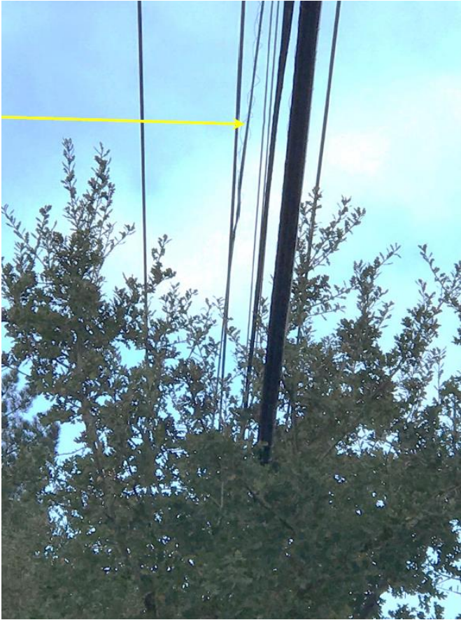
Figure 2. Photo showing broken/loose lash wire on communication cable.
