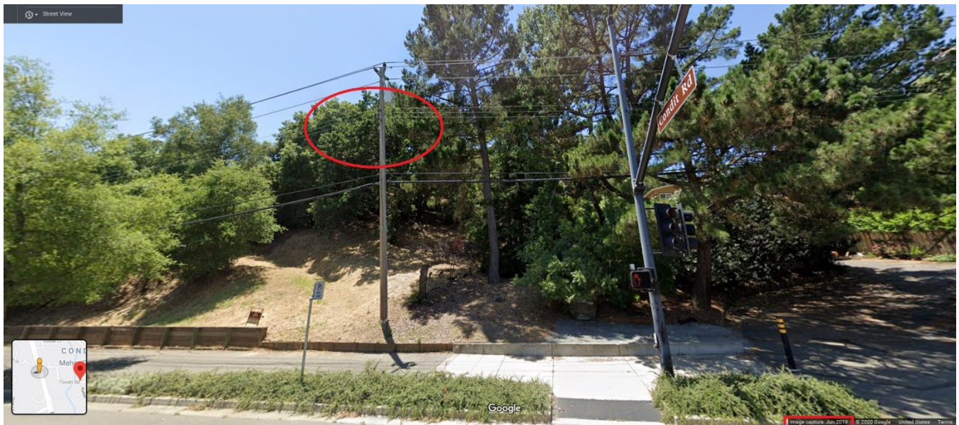
Figure 6. Google Street View image captured in June 2019 confirmed the communication cable had not yet been installed at the time. Source: Google Maps
