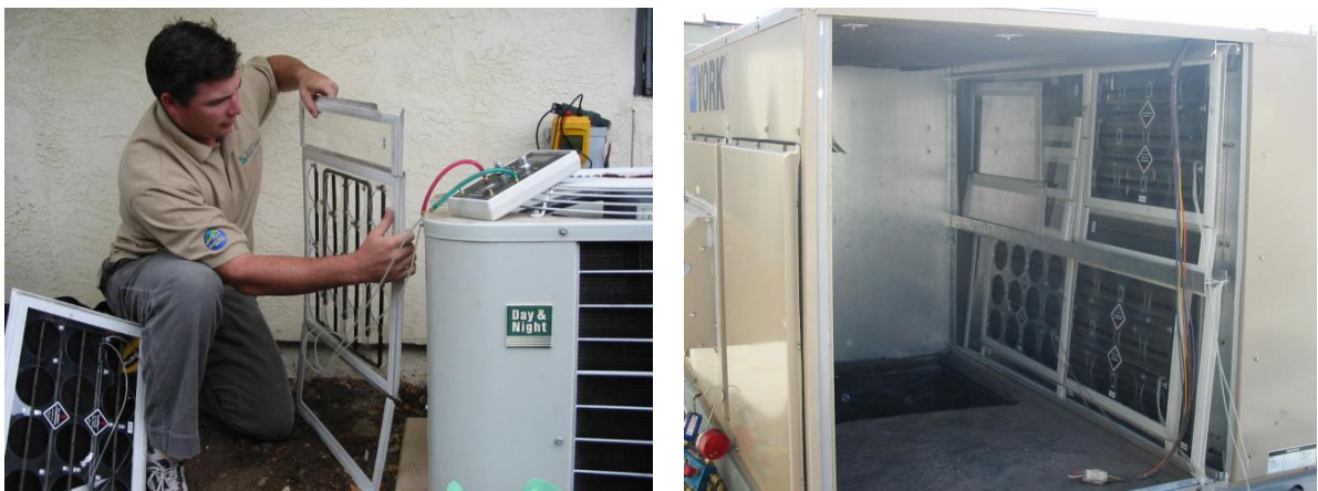
Figure 7.10: Airflow Measurements Using a Flow Grid
