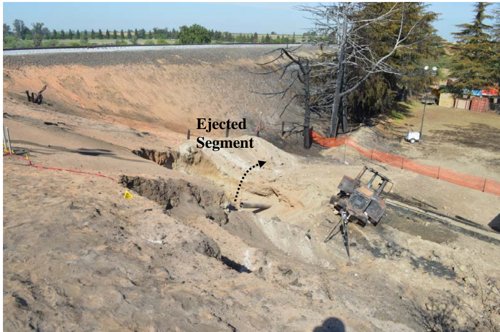
Figure 7. Photograph looking west toward the rupture crater from the top of the slope. The Ejected Segment is visible northwest of the crater.
