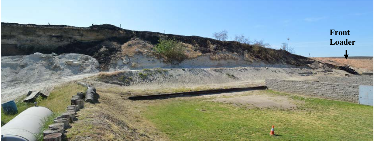
Figure 10. Photograph looking south from the shooting range toward the slope behind the range. This image, taken after the rupture occurred, shows the dirt road cut into the slope and extending from the near left toward the far right, where the front loader is visible.
