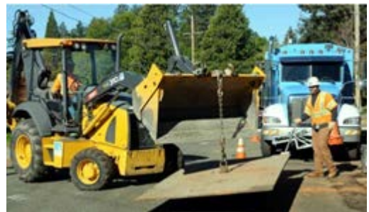
Figure 27 – PG&E's Super Crew at Work
