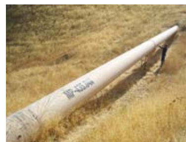
Figure 10 – Transmission Pipeline Span
