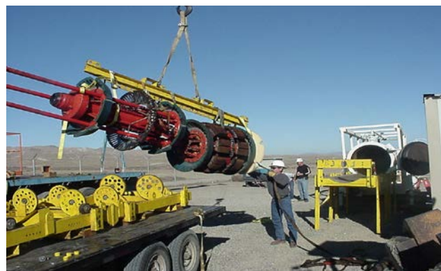
Figure 22 – A Magnetic Flux Leakage Tool or “Smart Pig” Being Loaded Into the Pipeline Launcher.
