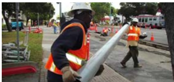
Figure 12 – Distribution Main Replacement Project
