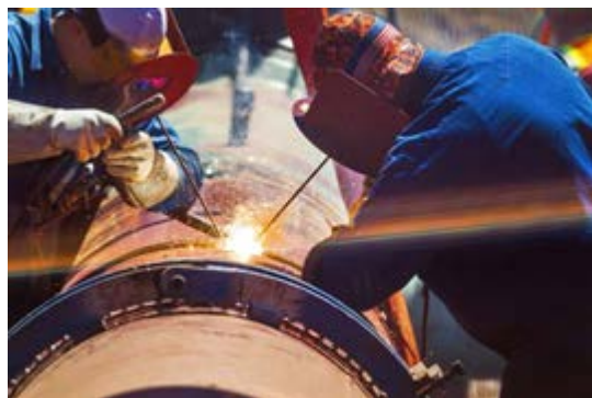
Figure 14 – Two PG&E Welders
