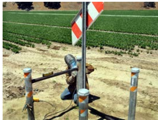
Figure 29 – Installing a Pipeline Marker and Physical Protection
