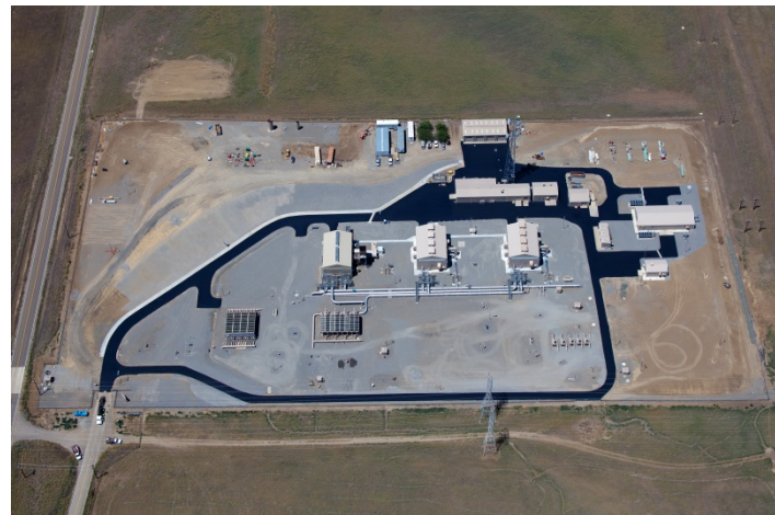
Figure 9 – PG&E’s Delevan Compressor Station
