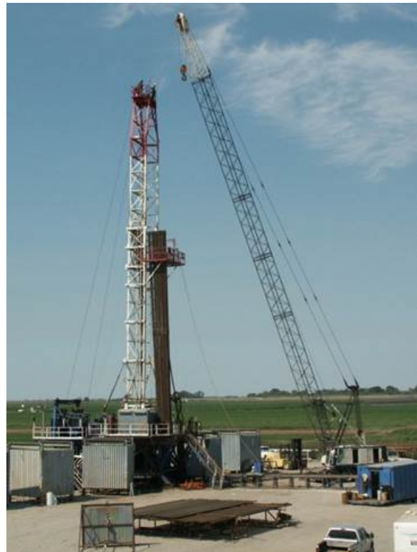
Figure 8 – Well Rework: Rig on Well
