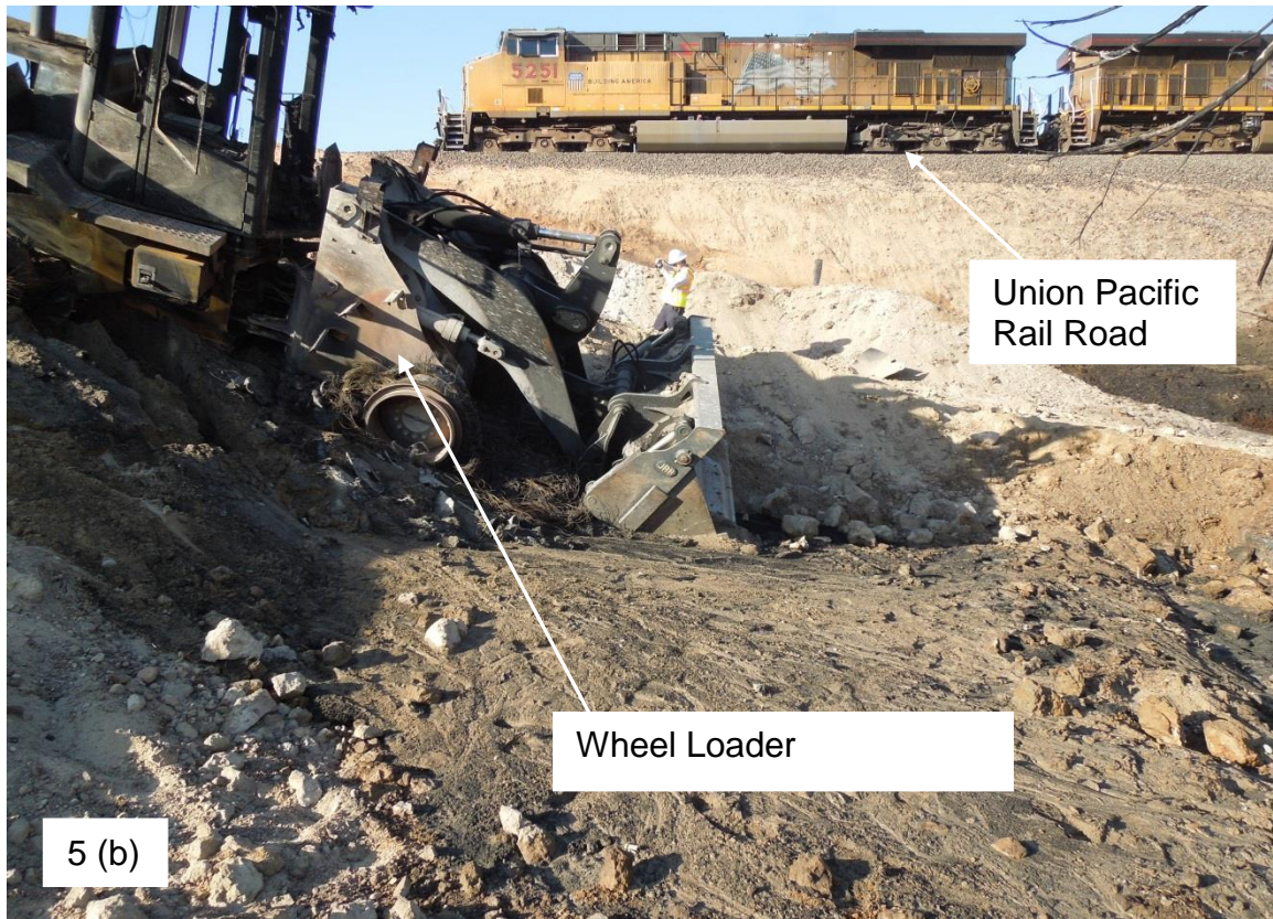
Figure 5: (a) Damaged Adjacent Union Pacific Railway Lines (b) the Wheel Loader
