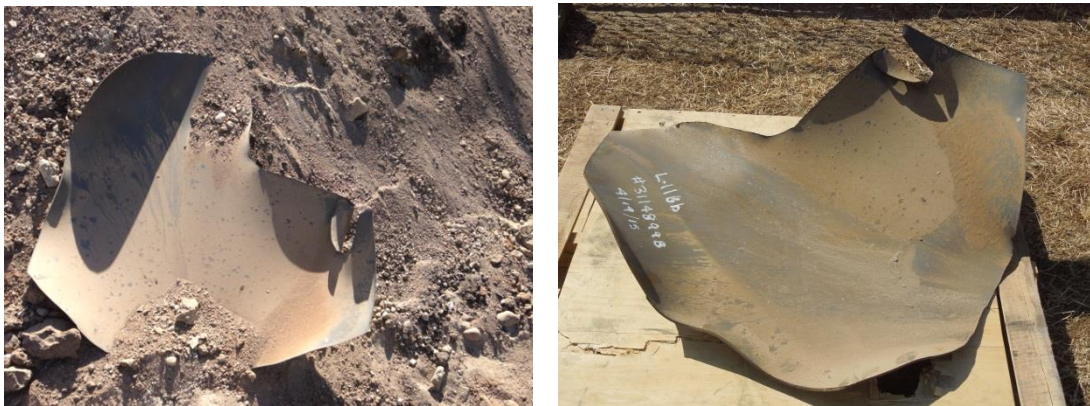
Figure 4: Ejected Portion of the Pipeline
