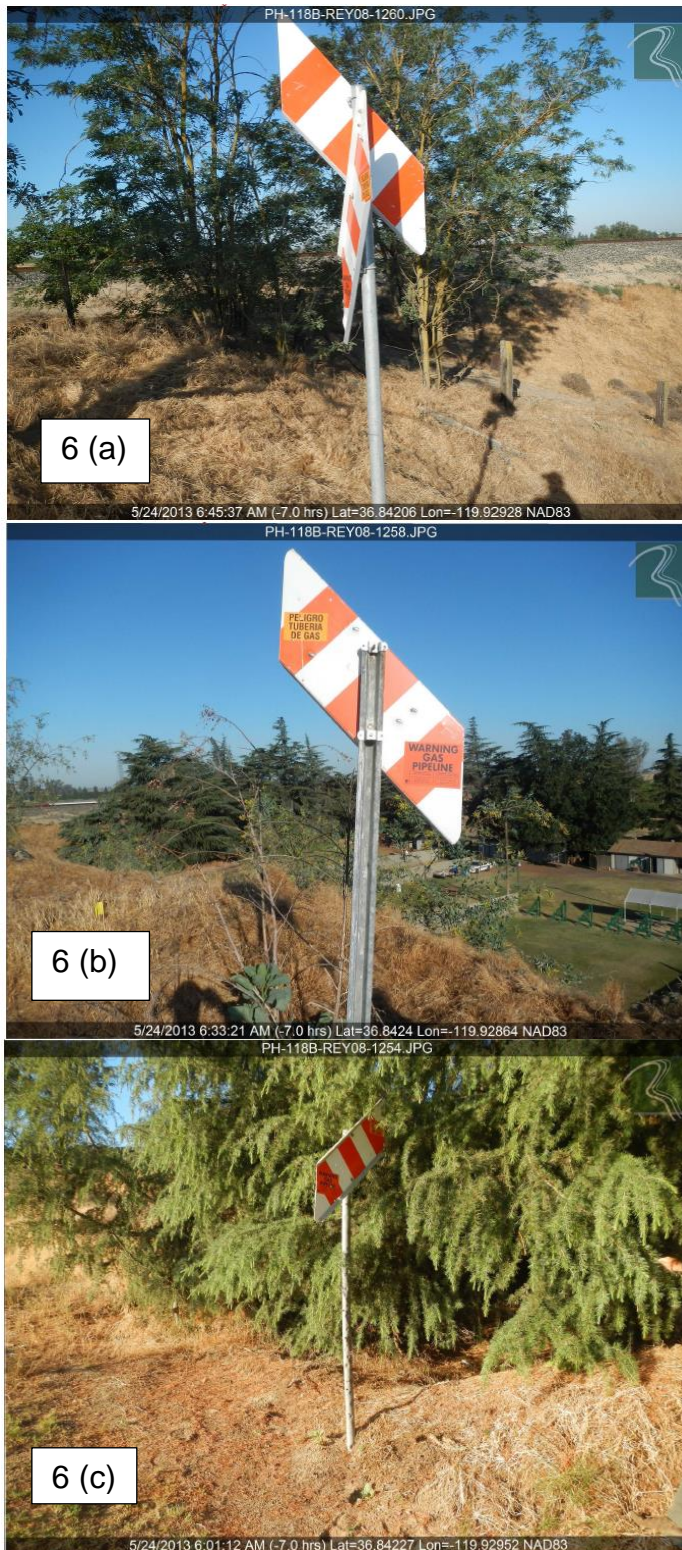
Figures 6 (a), (b), (c): Line markers and depth of cover in early 2013 at the incident location.
