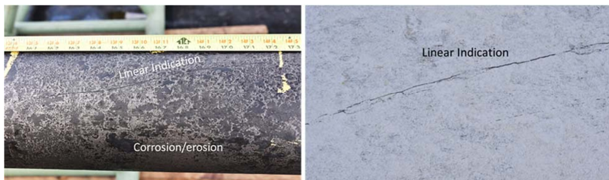
Figure 29: Example of oblique crack-like feature
