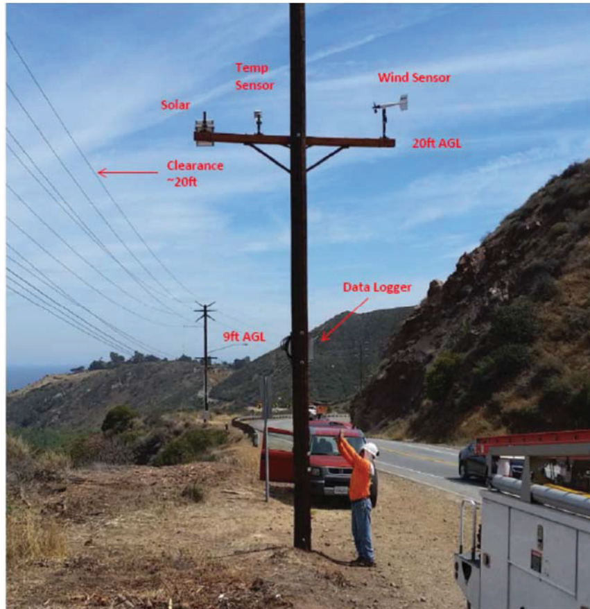
Figure 6. Station 3 looking South (courtesy Leidos).
