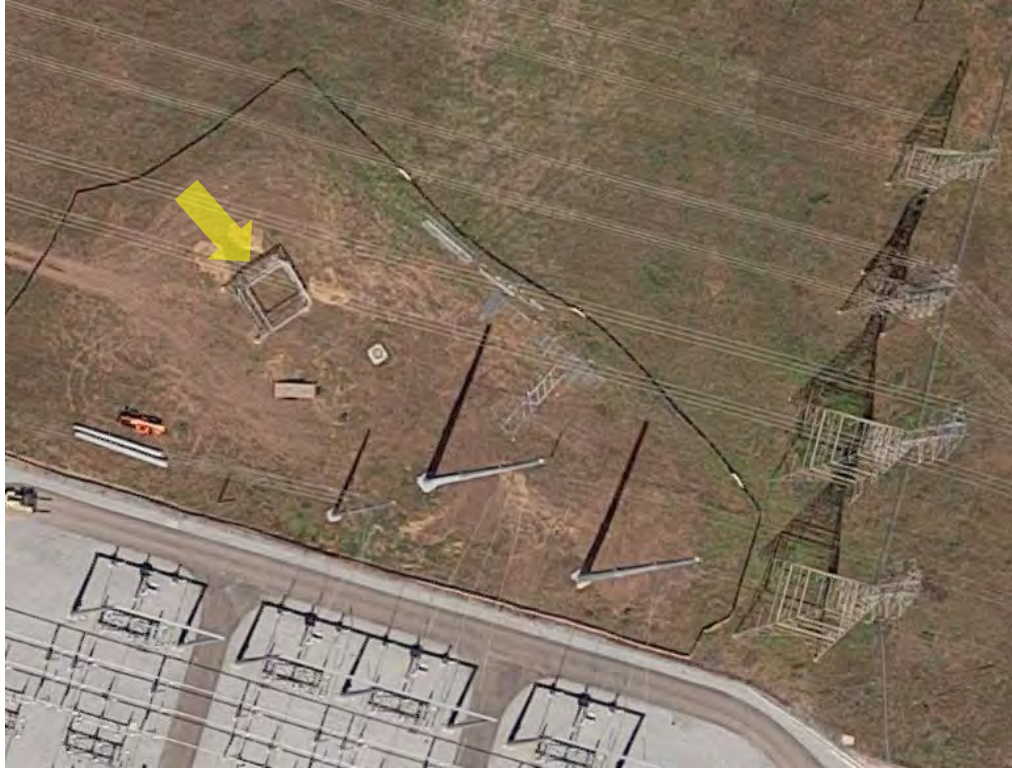
Figure 2. Overhead photo of subject tower, taken in April 2015 during tower construction. Tower base is visible in photo, identified with yellow arrow. (Google Earth)
