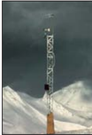
Meteorological conditions measured at Lake Louise, Alberta, Canada are tele-metered via phone-to-RF link to a base station.
