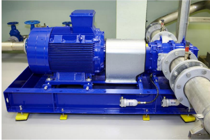
FIGURE A-56: TYPICAL PRESSURE REDUCTION TURBINE CONFIGURATION
