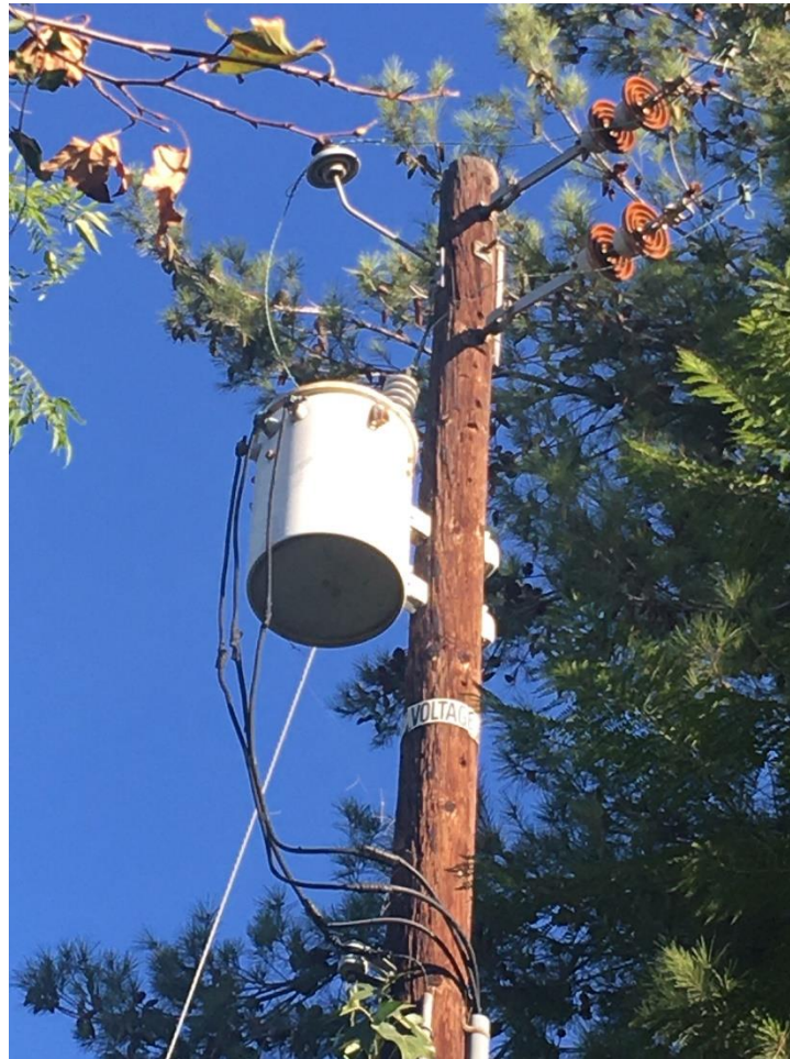
Circuit 305: Tree in Contact with P514617
