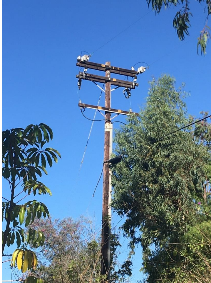
Circuit 305: Tree in Contact with P513641
