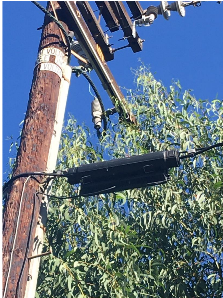
Circuit 305: Tree in Contact with P513641
