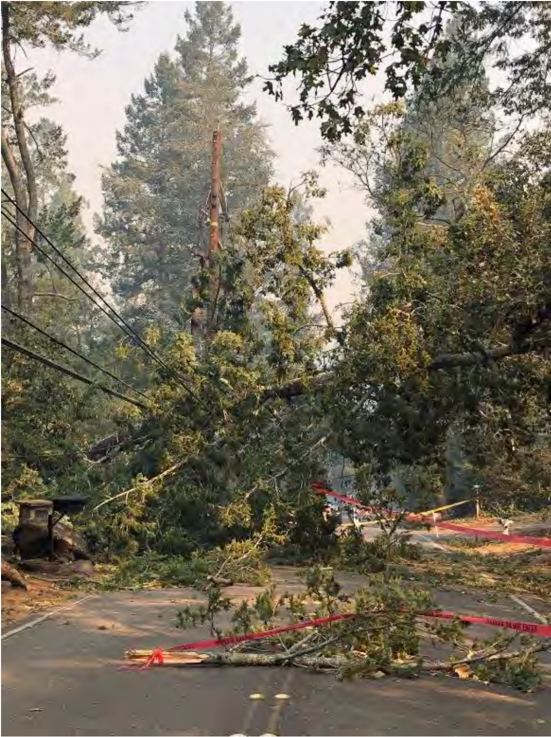
Figure 3: Tree failure, resulting in broken conductors in Santa Rosa, Sonoma County
