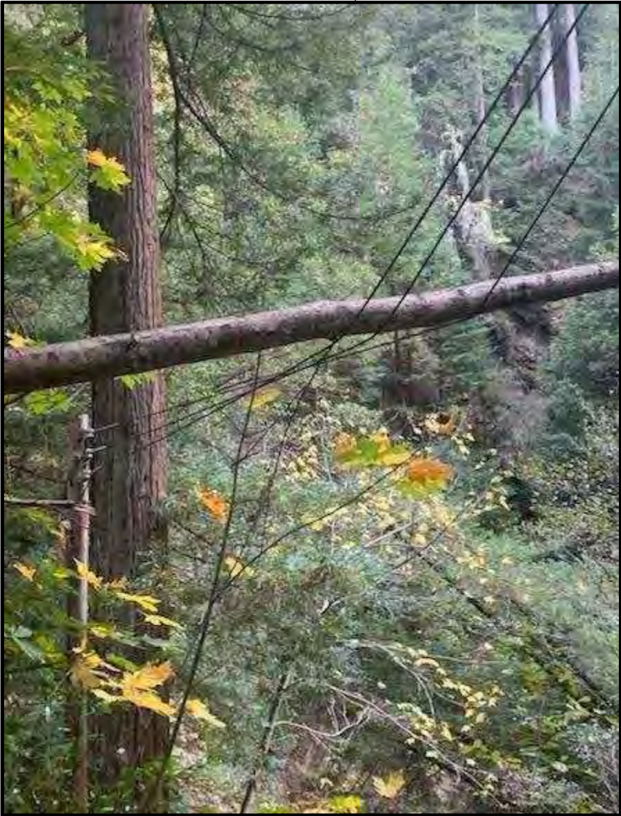
Figure 8: Tree fell onto conductors: Unincorporated area of Santa Cruz County
