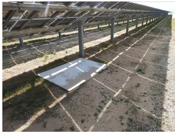
Sheets of plywood on ground creating tripping hazard.
