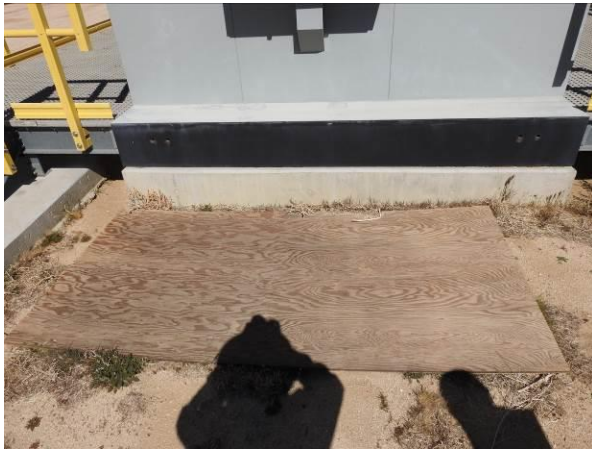
Sheets of plywood on ground creating tripping hazard.
