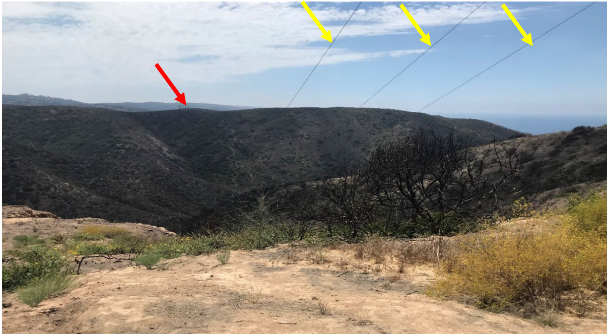
Figure 5. Photo of the three conductors (yellow arrows) spanning approximately 3650 feet east from Moro Ridge Road. The red arrow points to the three poles that support the conductors on the other side of the canyon near Boat Road.
