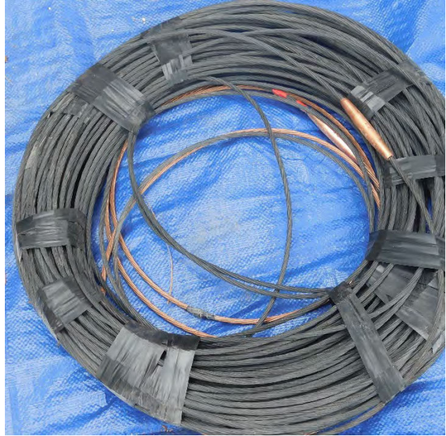
Figure 10: South phase conductor from the incident span
