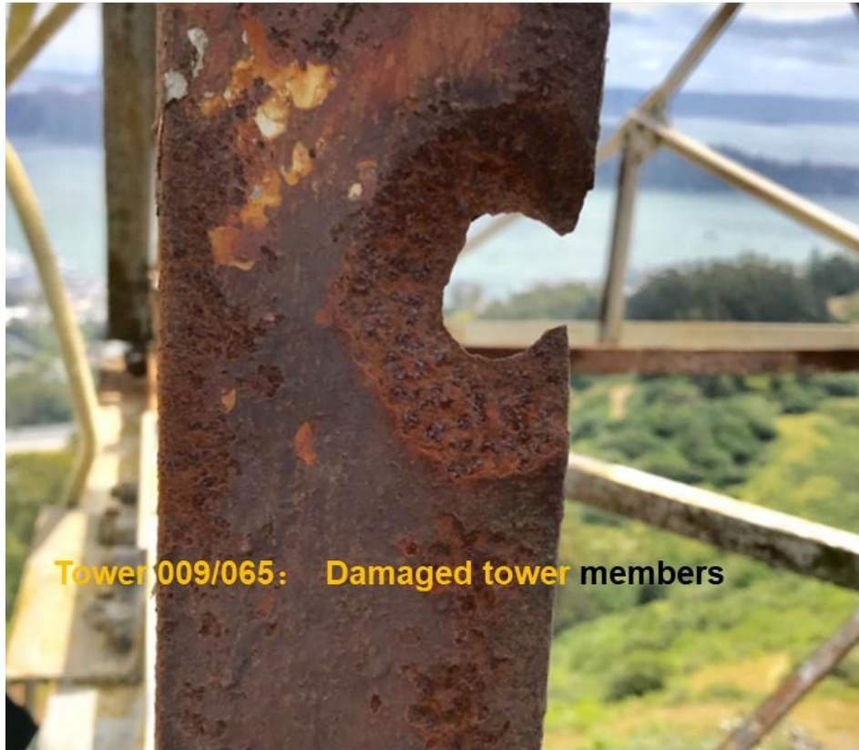
Figure 3: Identified Deficiencies (1)
