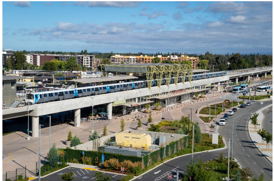
Berryessa Elevated Station
