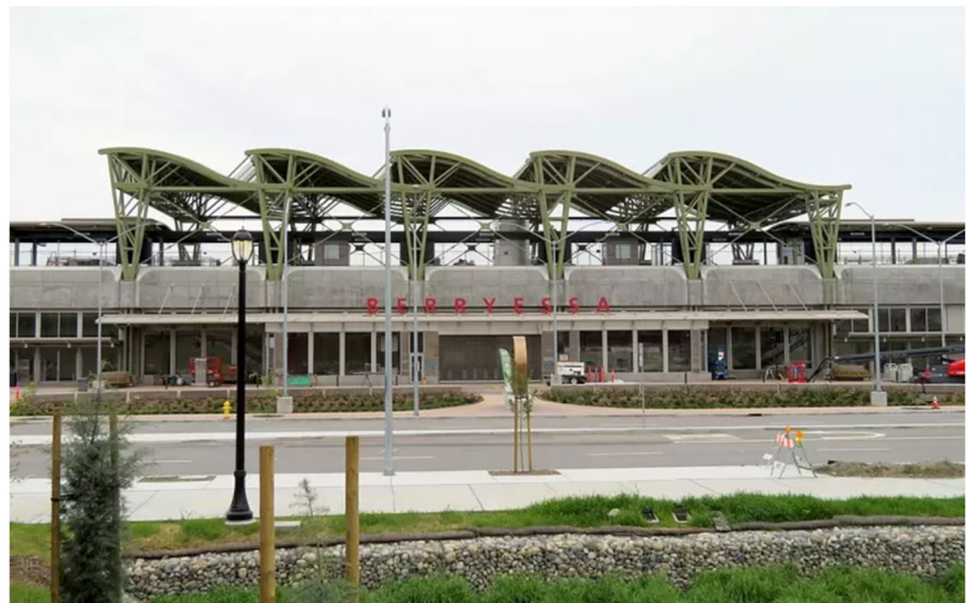
Berryessa Transit Center, connection between BART and VTA
