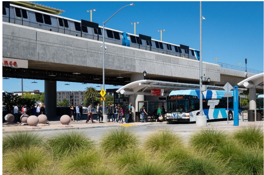
Berryessa Transit Center, connection between BART and VTA
