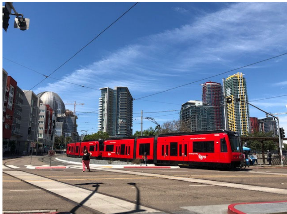
San Diego Trolley Light Rail Vehicle in Downtown San Diego
