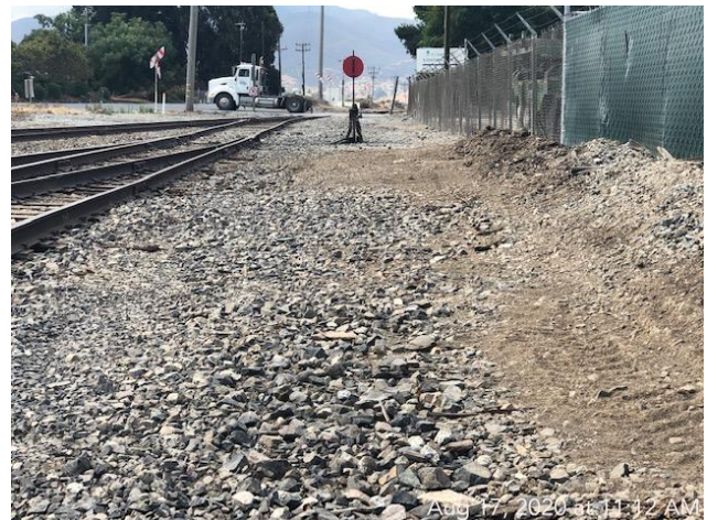
After: Graded walkway
