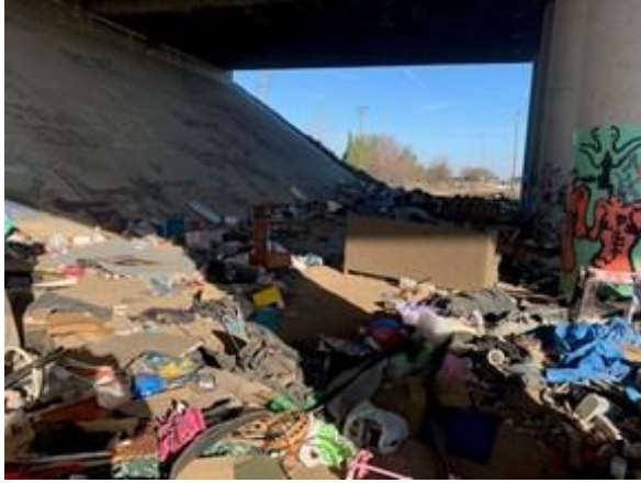
Before: Homeless encampment and debris on property
