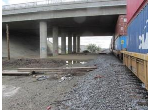
After: Encampment and debris removed from UPRR property
