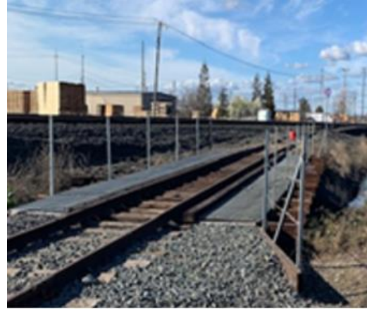
After: Vegetation cleared from bridge
