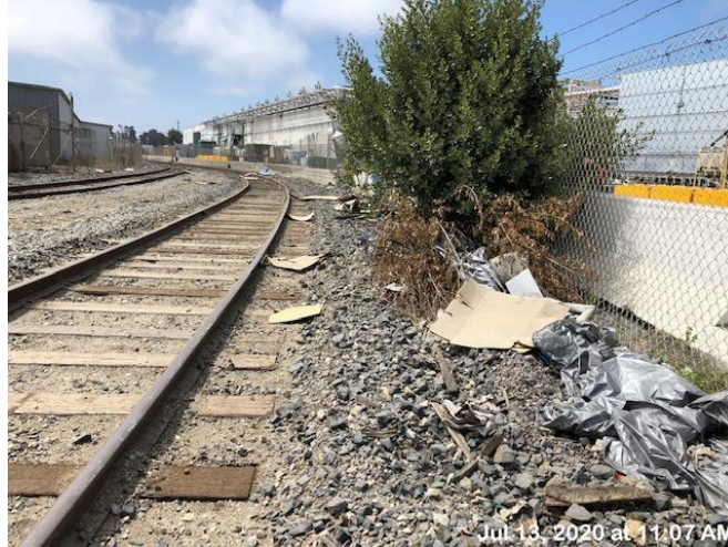
Before: Tree impeding minimum side clearance; debris on walkway
