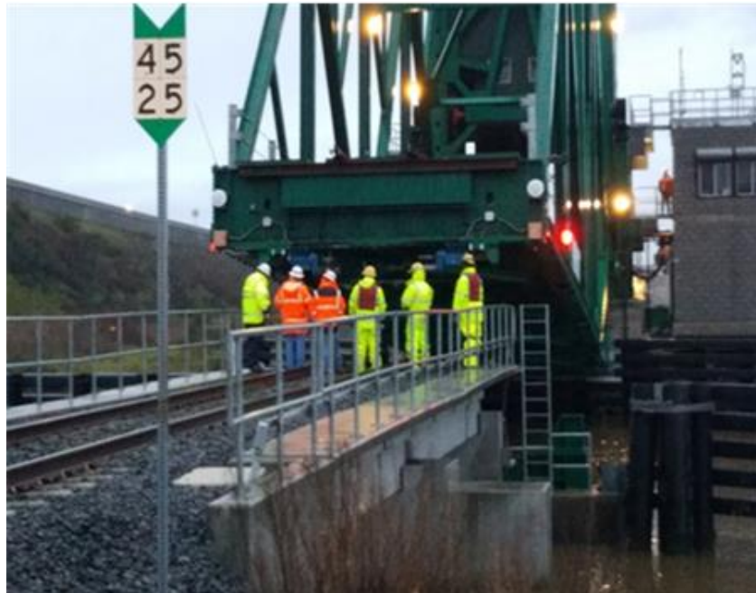
RSD and FRA Signal inspectors along with railroad company personnel conducting an inspection of a mainline bridge and signaling associated with bridge operation
