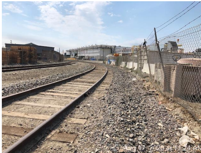
After: Tree and debris removed
