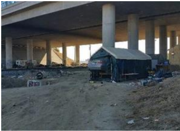
Before: Homeless encampment and debris near UPRR 8 Mile location
