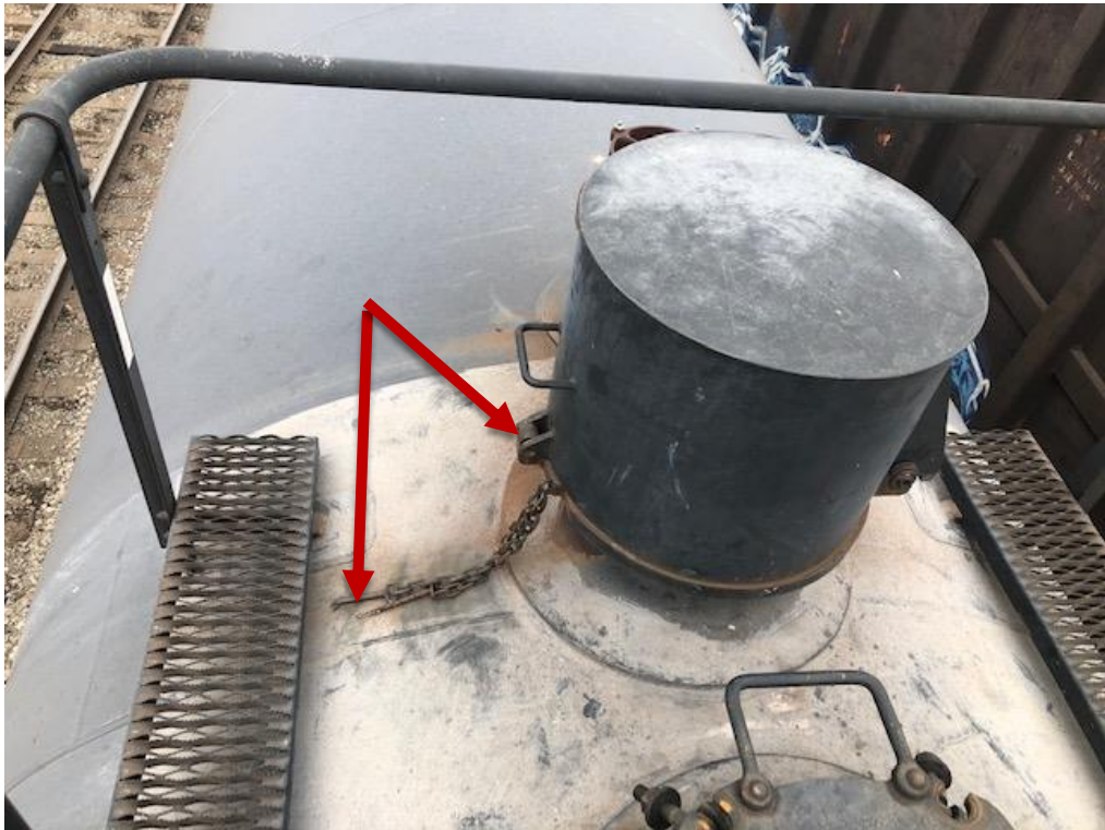
Protective housing pin not properly placed for securement
