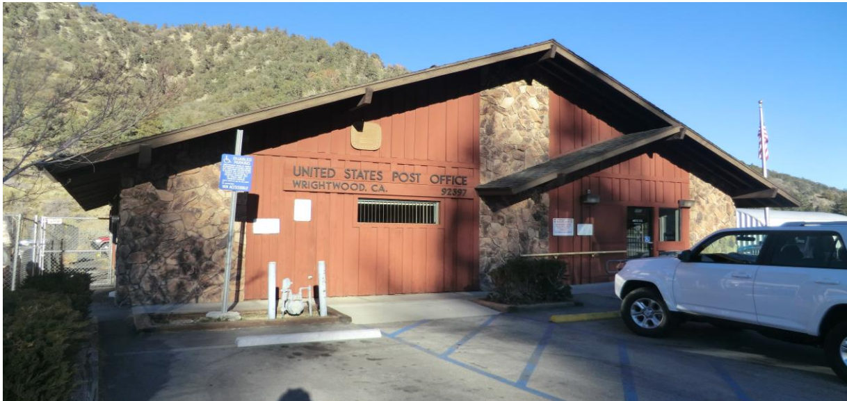
United States Post Office in Wrightwood, CA, project funded by CASF
