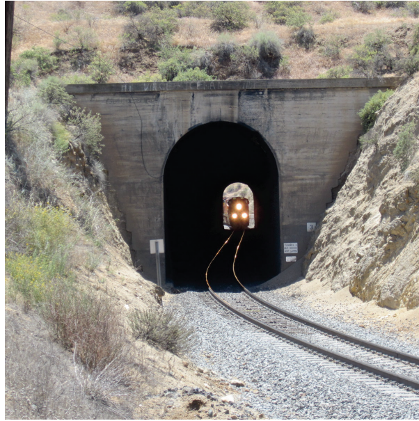
Westbound freight train entering Tunnel #3 in Tehachapi Pass (Local Safety Hazard Site No.16)
