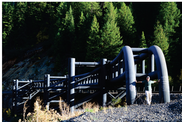
Derailment barrier on the Cantara Loop bridge. 13
