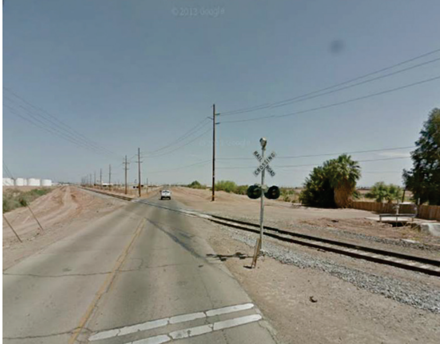
North 8th St. /Clark Rd. railroad crossing, view from North 8th St. side of crossing. The railroad crossing blind spot is located on the right
