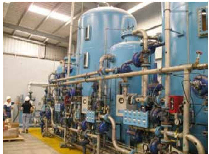
CPUC staff conducting an inspection of power plant equipment
