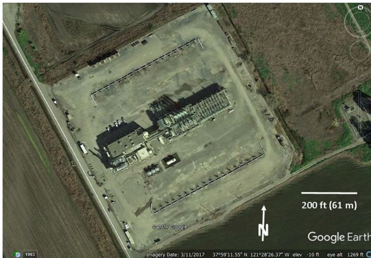
Figure 1.2-30. Aerial view of the McDonald Island Turner Cut station showing control room (SW end of central structure) and gas processing facilities (NE end of central structure) and two WSW-ENE trending lines of wells on 25 ft (7.6 m) spacing on either side (north and south) of the central structure.
