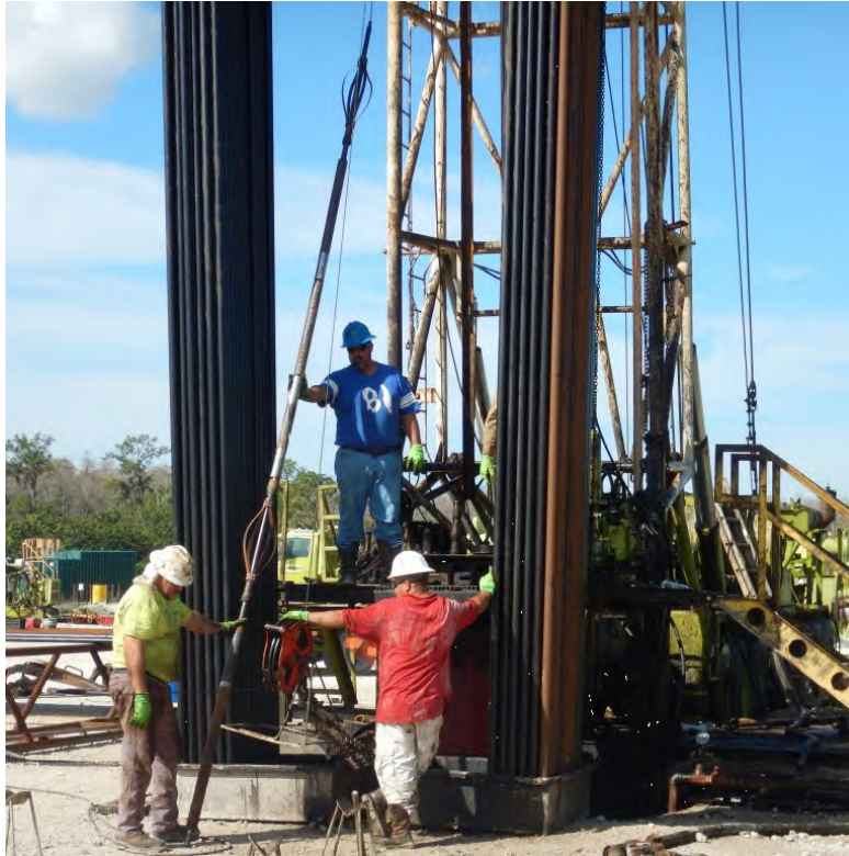
Figure 1.3-2. Example of a well work-over underway (Source: ALL Consulting, LLC, 2016).
