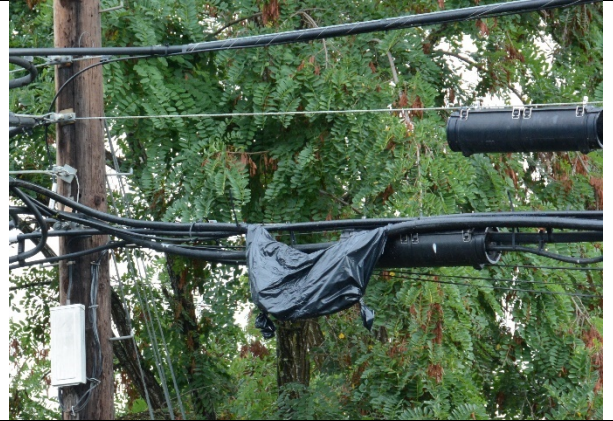
Splice location with plastic cover
