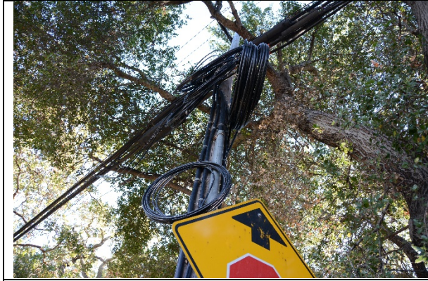
Fiber build-out in progress
