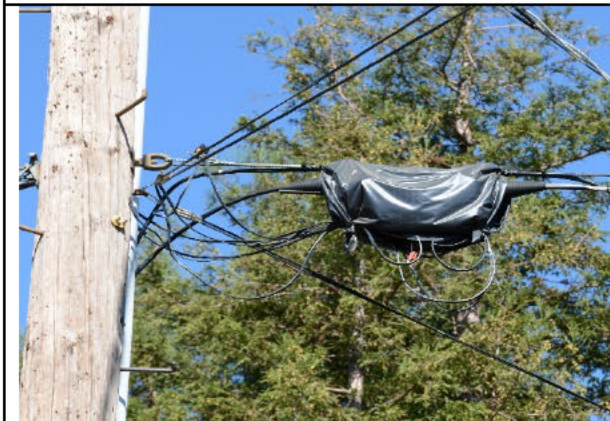
Splice wrapped in plastic drapery (Nicolaus)
