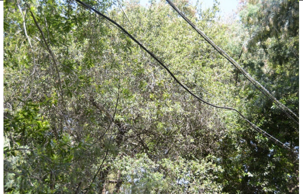
Cables de-lashed from support strand
