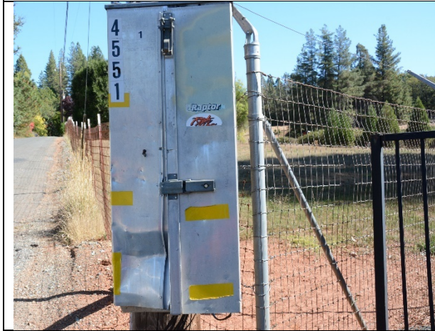
Dented cross-connect box
