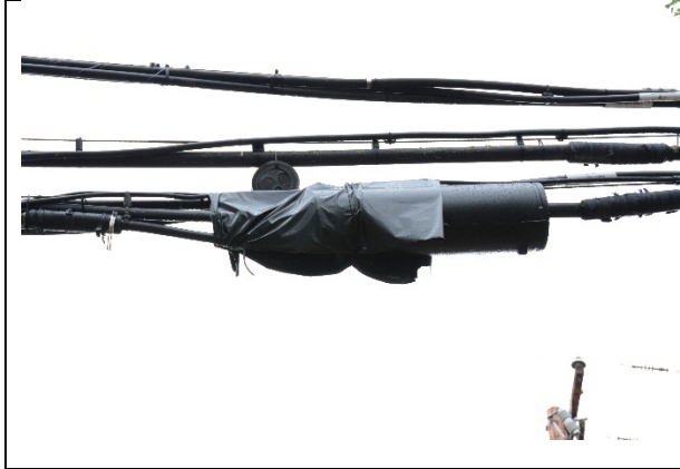
Temporary splice closure in Boonville
