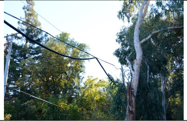
Cable de-lashed from support strand
